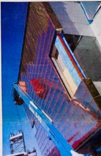
Dave McKnight, of Dave McKnight Construction of Welland, Ont., installs copper panels on the new city hall in Welland on Thursday.
